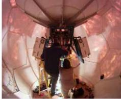
Technicians work to repair the satellite antenna in the VSAT dome. Image courtesy of NOAA Okeanos Explorer Program. http://oceanexplorer.noaa.gov/okeanos/explorations/ex1103/logs/hires/dome\_hires.jpq
