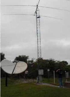
Note that the antenna is mounted on TOP of the tower. Image credit: NOAA. http://www.srh.noaa.gov/images/mlb/032v2.JPG
